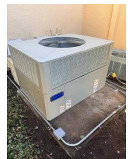
American Standard 5 Ton Package Unit Replacement
